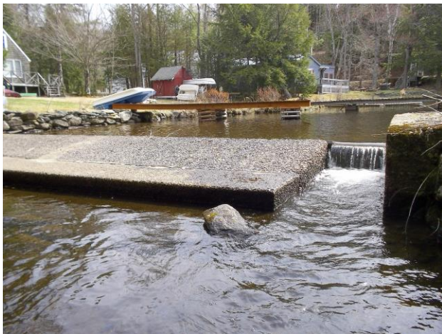
Check out the CLA dam at the east end of the lake. Photo by Tim Perry
